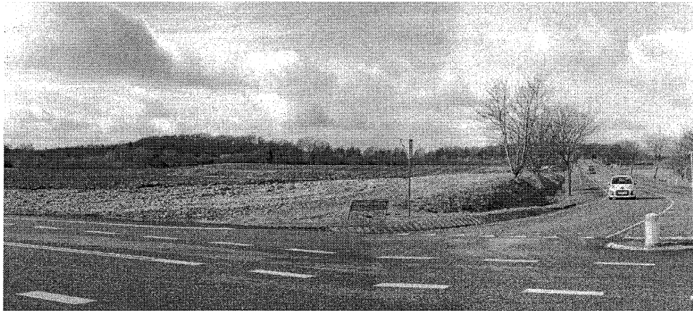
Figure 3-1. The location of the substation as seen from the east at the intersection of Slimmingevej and Vordingborgvej, as the area appears today. The landscape is defined by open areas and woods towards the horizon.
