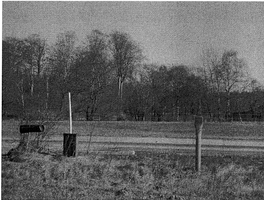
Figure 3-5. An example of a marker indicating a cable buried underground.
