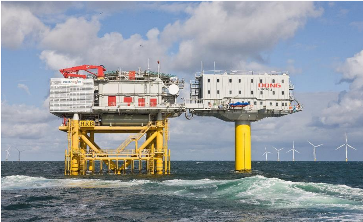
Figure 3-8 Example of an accommodation platform (right) at Horns Rev 2 sea-based wind farm, with a substation located adjacent (left). The accommodation platform is placed on a monopile foundation while the substation has a jacket foundation.
