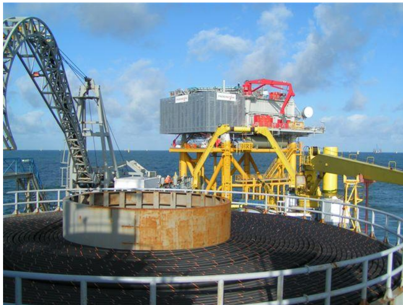
Figure 4-2 Installation of cables from cable-laying vessel at Anholt (Photo: Ramboll).
