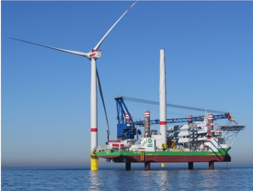
Figure 15. Installation of a wind turbine using a jack-up vessel. Source: COWI
